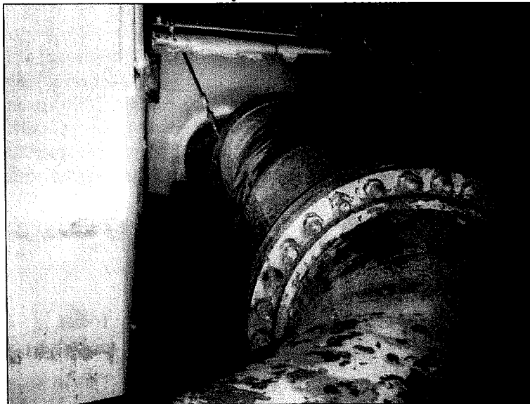
Photograph 5 (Longitudinal View of the 30" diameter intake line At the Westerly foundation wall.)
